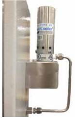
Figure 2-58: Thermostat Inside the Touch Screen Enclosure
